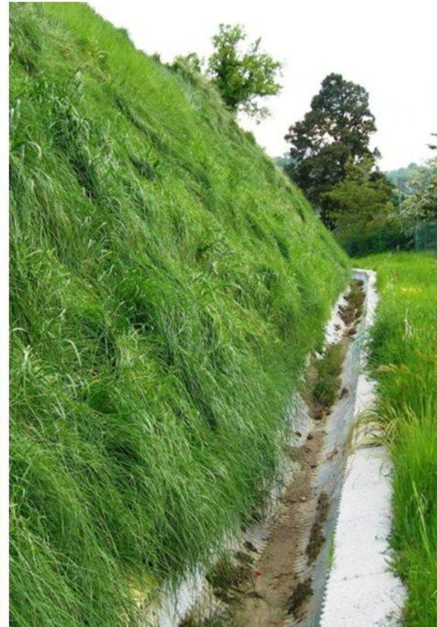
b) clean drains
