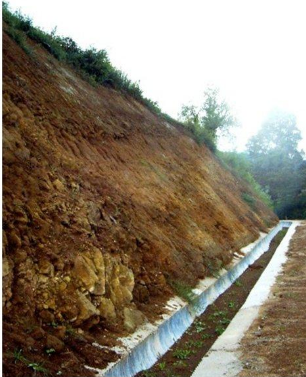
a) clogged drains
